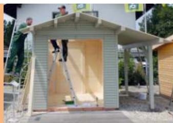
Constructing the roof boarding
