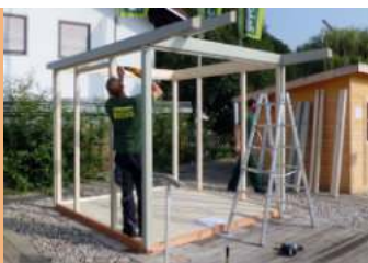
Assembling the skeletal structure
