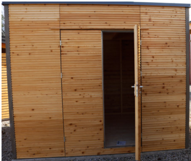
No adjustable hinges on outward-opening doors, only on inward-opening flush-to-wall closed doors.
