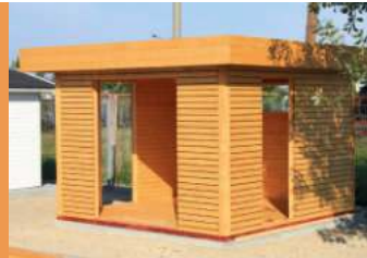
Roof boarding and wall cladding
