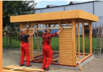
Mounting the rhombus cladding
