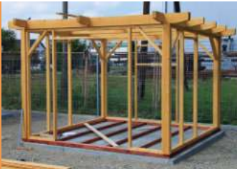
Timber frame construction
