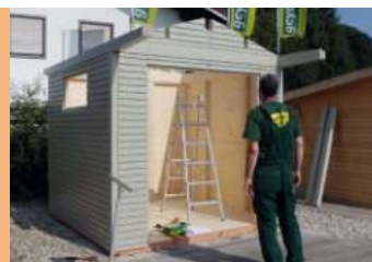
Inserting the fully assembled wall and gable elements
